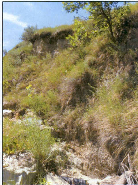
Photograph 12. 12-foot-tall embankment along western margin of fill area. CMP drainpipe at bottom of photo. View to south.
